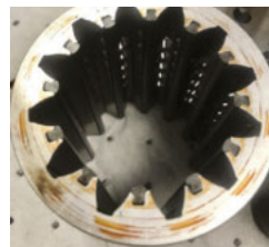
Component inspection 1-month after DECON showed significant amounts of deposits had dissolved.
